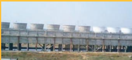
SUPER THERMAL POWER PROJECT AT NAGPUR, MAHARASHTRA
